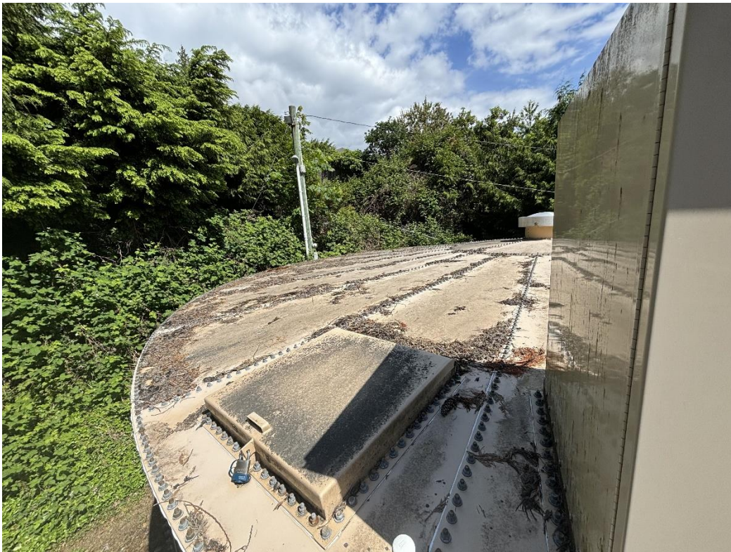
Figure 16 North Tank Roof Access
