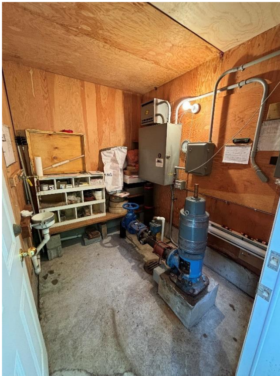
Figure 11 South Well House Interior
