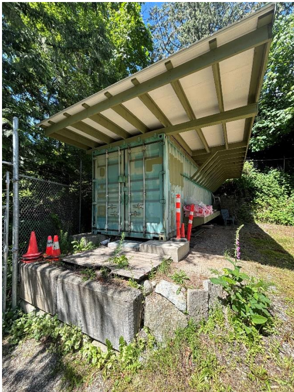
Figure 23 Structure Housing Controls and Electrical Onsite
