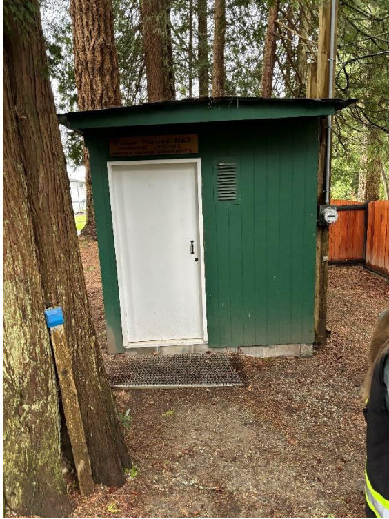
Figure 1 North Well House
