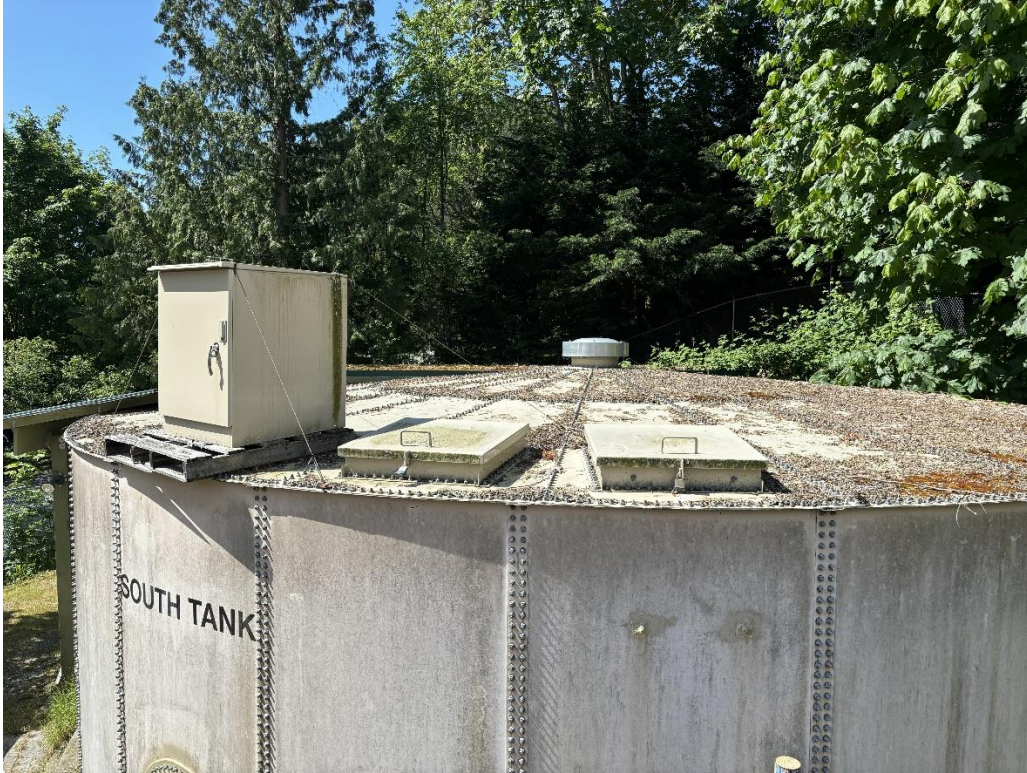
Figure 15 South Tank Roof Access
