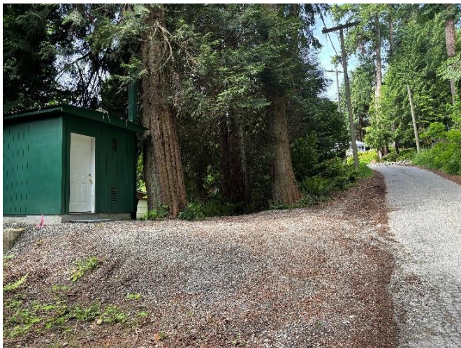
Figure 7 South Well House Site Access
