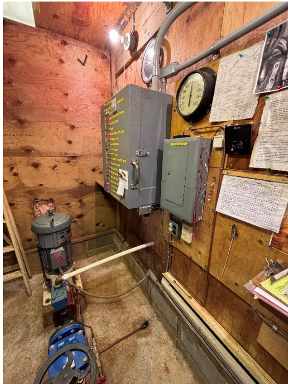
Figure 4 North Well House Interior
