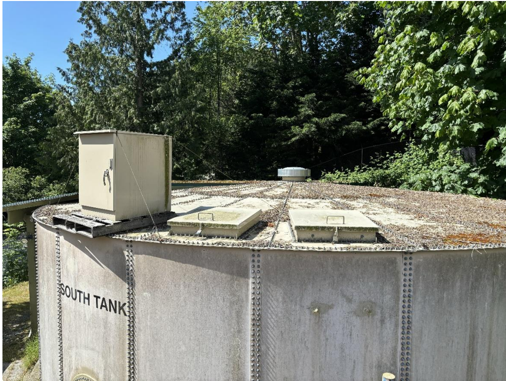
Figure 15 South Tank Roof Access
