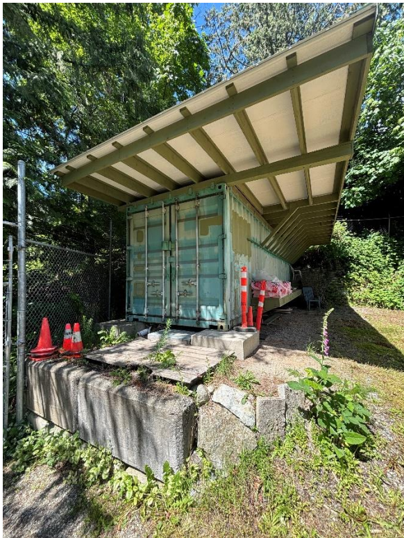
Figure 23 Structure Housing Controls and Electrical Onsite
