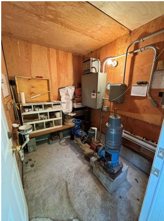
Figure 11 South Well House Interior
