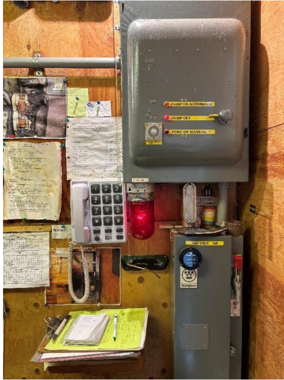
Figure 2 North Well House Interior
