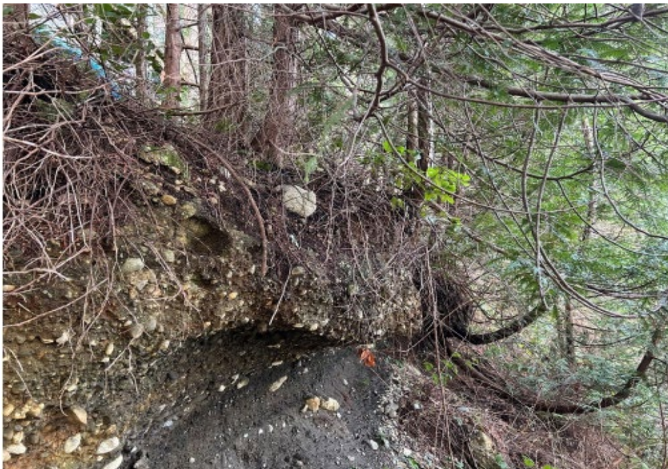
Photo 2 – Closer view of unstable overhanging materials with overlying vegetation.
