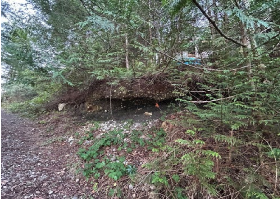
Photo 1 – Immediate Hazard. Unstable overhanging materials with overlying vegetation. 488 Collingwood in background.
