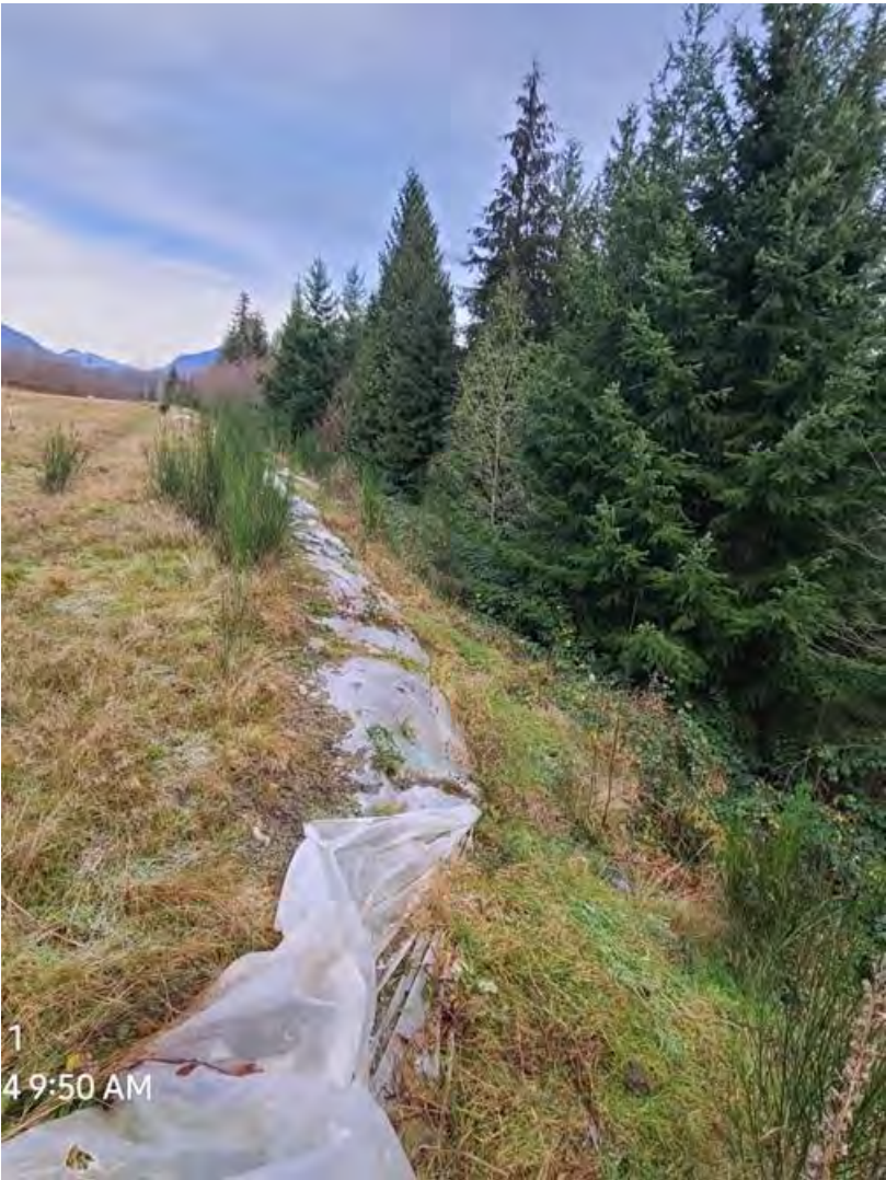
Figure 4. East-facing retaining slope of fill area. Plastic sheeting installed along edge of fill to mitigate sloughing of soil into adjacent parcel. Photograph facing north.
