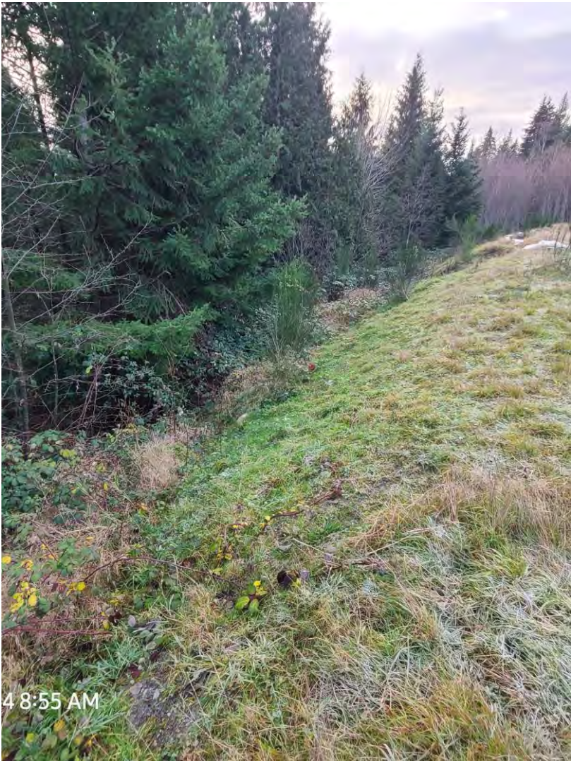
Figure 5. East-facing retaining slope of fill area. Edge of the fill is strongly (>25%) sloped and vegetated with grasses, blackberry and Scotch broom. Photograph facing south.
