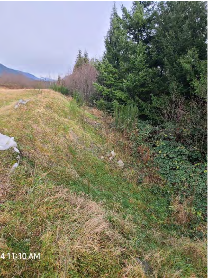
Figure 6. East-facing retaining slope of fill area. Stable slope with minor sloughing observed.
