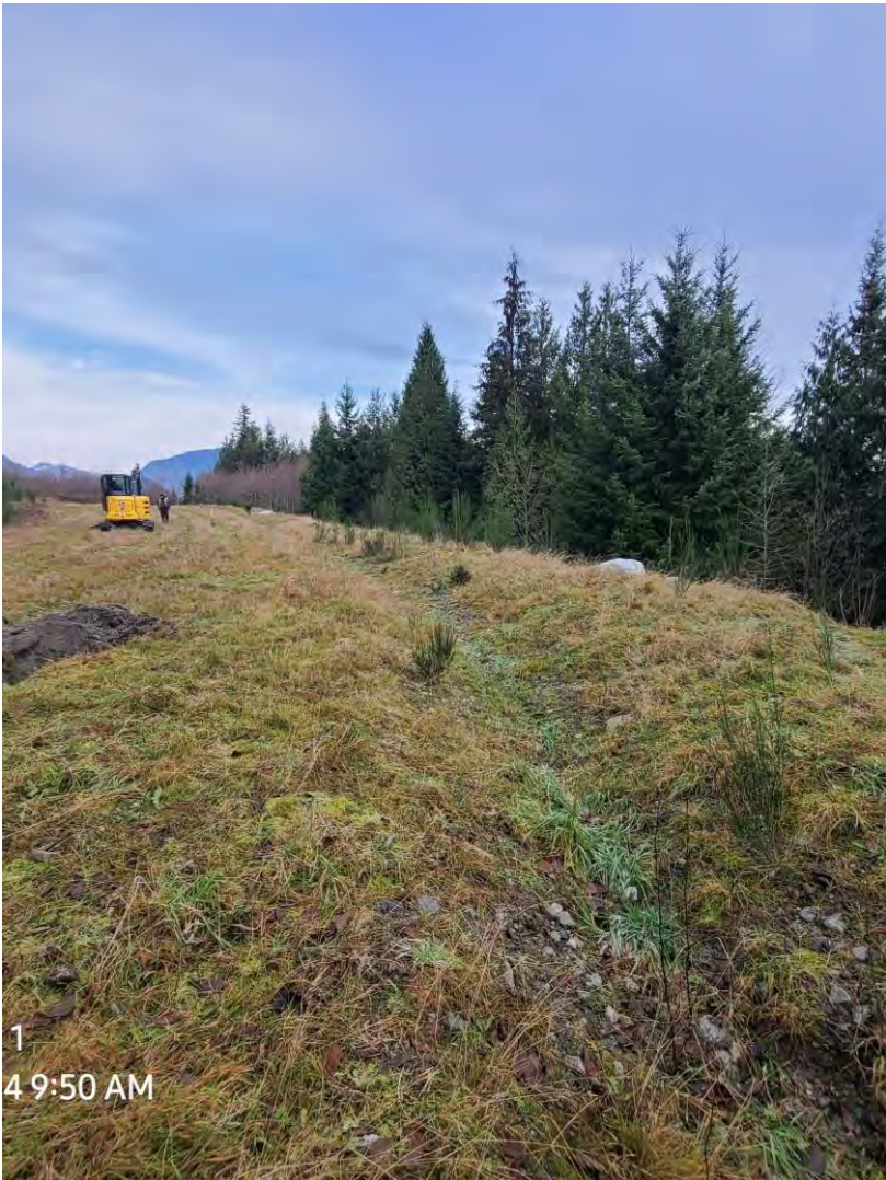
Figure 8. Terminus of drainage ditch along eastern edge of fill area. Drainage is directed towards a wooded area along the southern edge of the Site. Photograph facing north.
