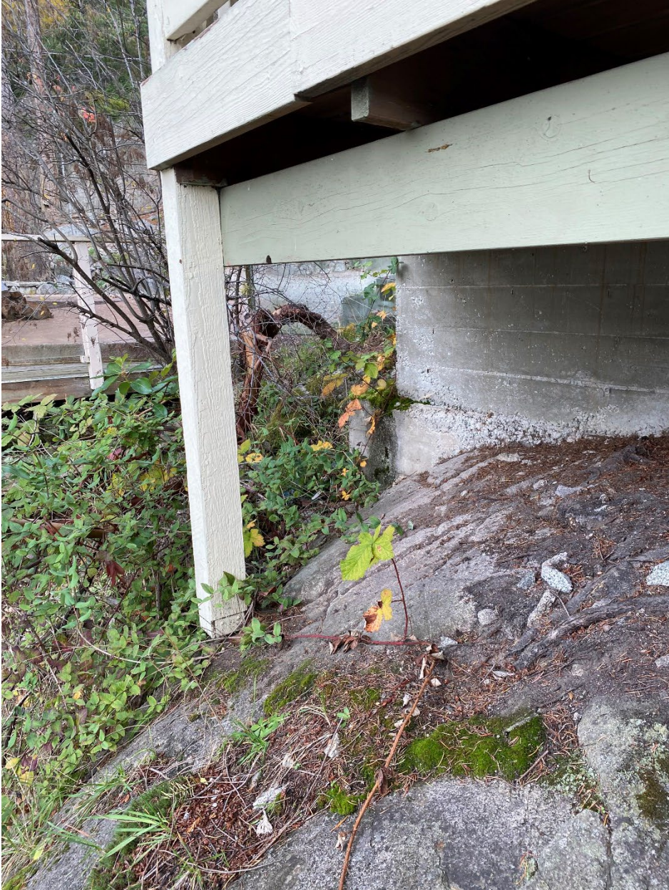
Figure 3: Existing Deck posts on bedrock
