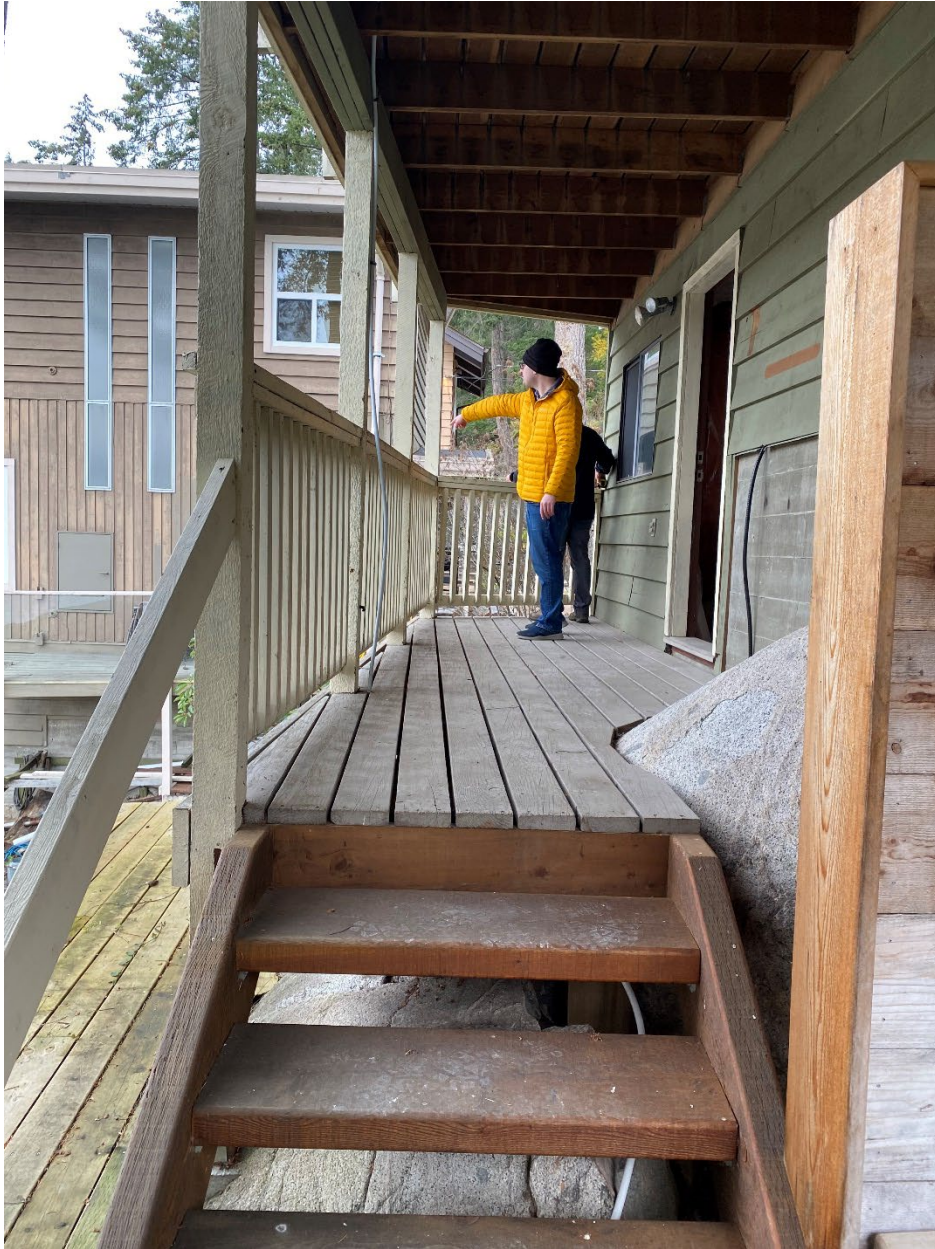
Figure 1: Lower Deck to be replaced
