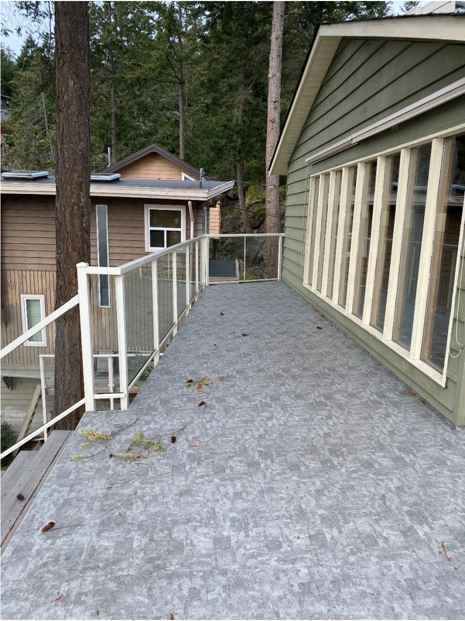
Figure 2: Upper deck to be replaced
