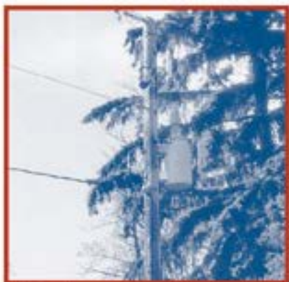
Contact utility companies for clearing of vegetation under overhead electrical installations.
